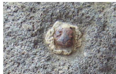
Fig. 14. Iron pivot with lead bonding in a meta (3M).
