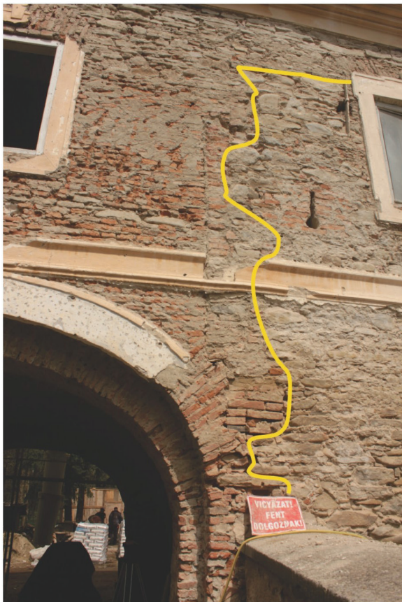
Plate IV. 1. Western side of the northern wing: 1. Defensive wall; 2. Walled-up vaulted passage; 3. Southern wall of the palace section built in the second half of the 16th century; 2. Original masonry of the gate tower with keyhole-shaped loop hole and later adjoining wall sections; 3. Trench 21: infilling of the moat.
